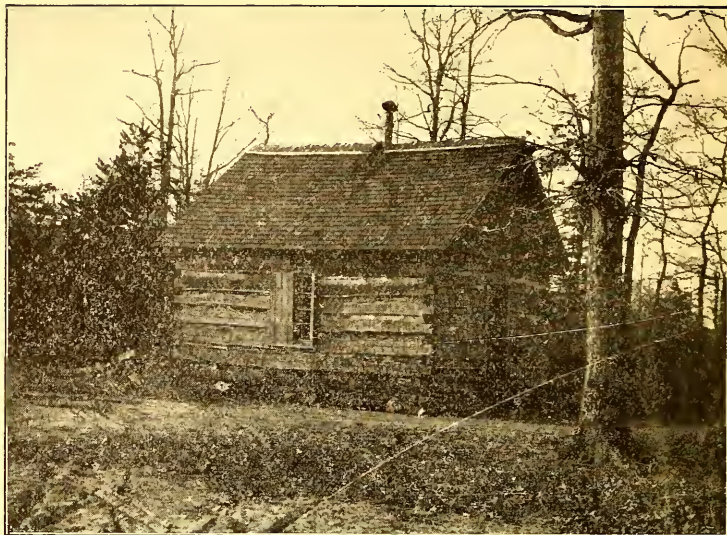
WILLIAMSBURG, No. 2, ROCKINGHAM COUNTY (OLD).
